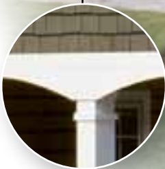
Restoration Millwork Wrapped Column and Routed Trimboard
